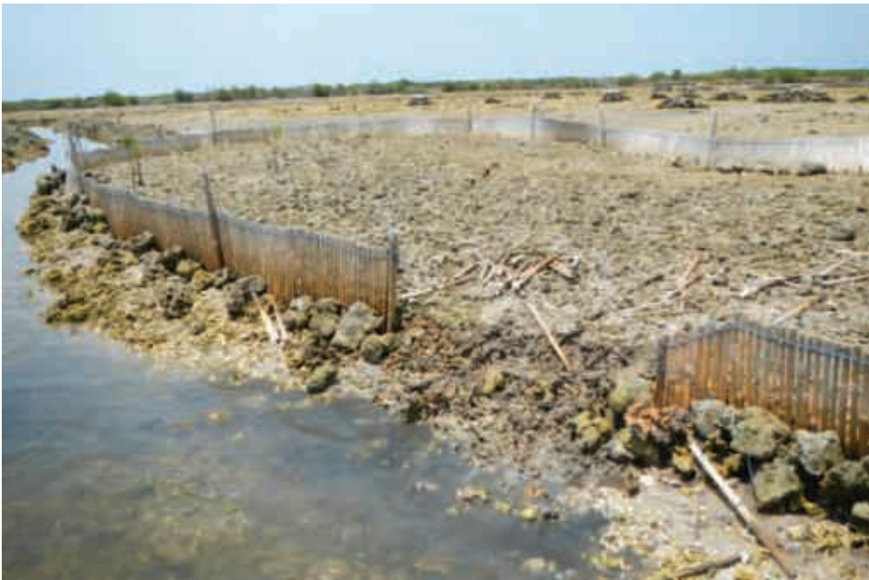
Fig 8.14 A mounded area (elevated 20 cm above pond bottom) with temporary bamboo fence next to a hand dug tidal channel. Tompotana, South Sulawesi, Indonesia.
