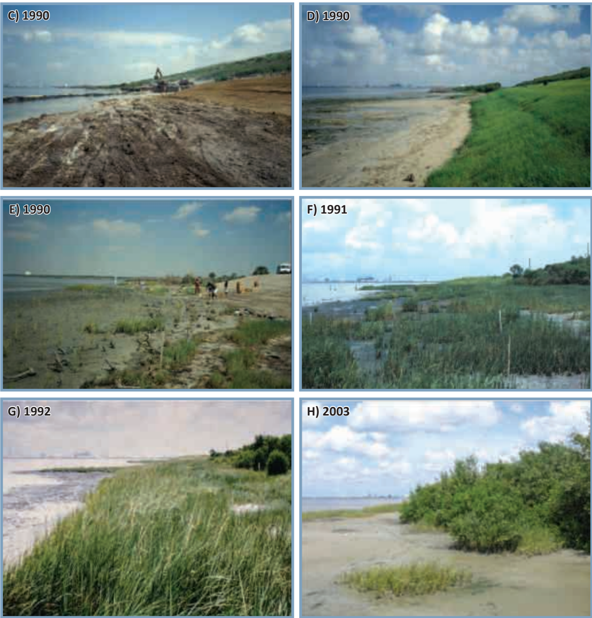
Fig: 8.29: Vertical erosion bluffs at the site indicated severe erosion (A - opposite page). The erosion bluff was cut back and re-graded to create a stabilized slope (B-C). Terrestrial grass was planted to hold the upper slope, followed by marine tolerant smooth cord-grass which stabilized the intertidal substrate (D-G). Thirteen years after the intervention, mangroves are shown, having succeeded the marine tolerant grass. Shoreline erosion at this site is no longer an issue.
