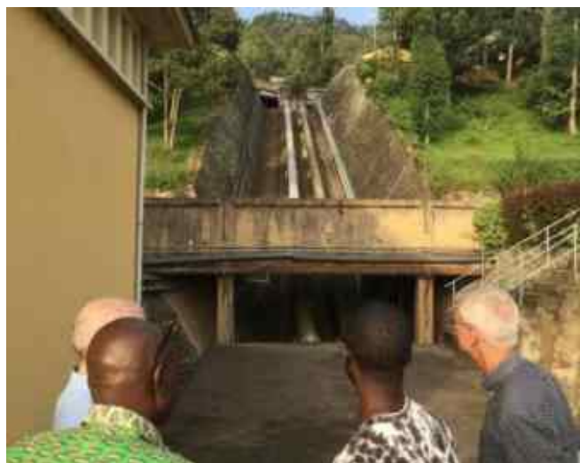
Rwanda: Tubes carrying water to a power plant. When sand-mining causes heavy siltation of this water, the power plant is regularly shut down to clean the turbines. The ROAM process can help stakeholders identify better siltation capture solutions upstream, allowing for a more stable electric power source. Photo credit: Mirjam Kuzee.
